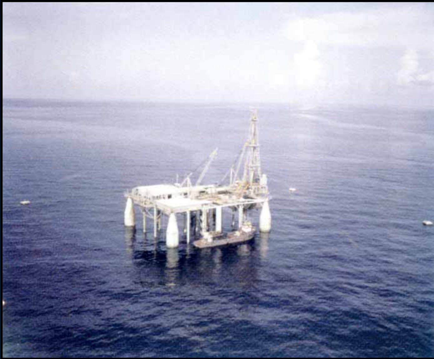
World's First Semisubmersible Bluewater I
