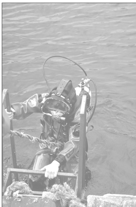
Figure 4: A diver entering the water via a ladder. Note how the tender is holding the umbilical and is supporting the divers weight
